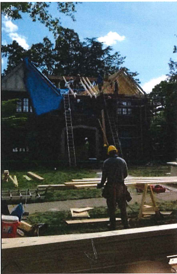
Roof Line and structure damage from front right and left original gables to rear of home addition. Approximate length of damage 84ft. Repairs to home's roof line so structure could be protected from the weather. Damage to the roof lines, boxing, gables, brick veneer and limestone appointments, slate roofing, tudor siding and stucco work, hvac units, and other related features.
