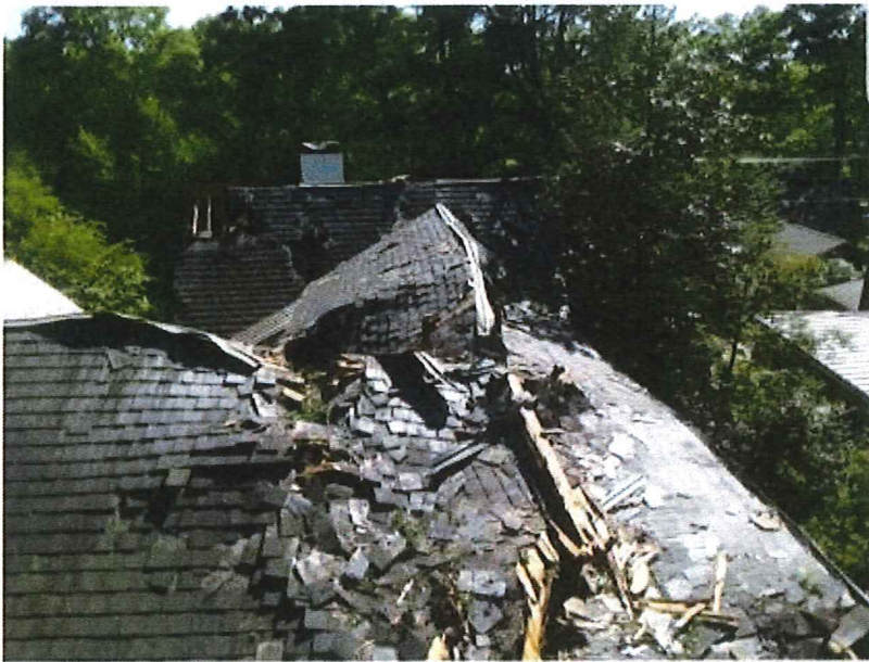
Roof Line and structure damage from front right and left original gables to rear of home addition. Approximate length of damage 84ft. Repairs to home's roof line so structure could be protected from the weather. Damage to the roof lines, boxing, gables, brick veneer and limestone appointments, slate roofing, tudor siding and stucco work, hvac units, and other related features.
